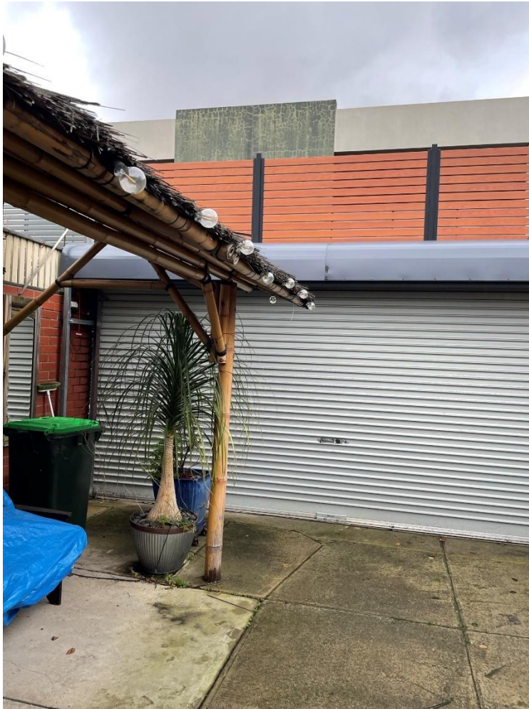
Photo 3.9 - Looking west from the rear yard of subject site
